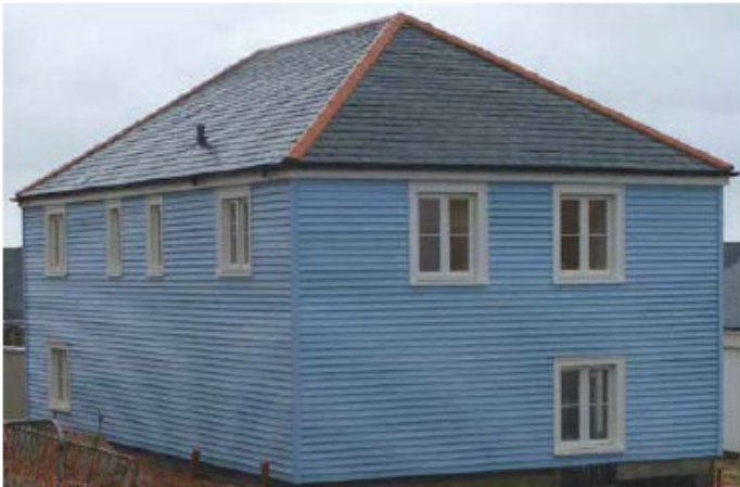
Painted timber building
